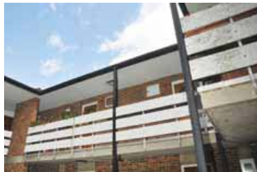
Figure 18 AIB exterior panel on open walkway
