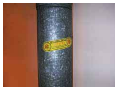
Figure 43 Metal clad gas flue containing chrysotile lining
