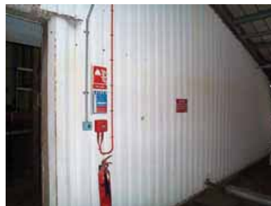
Figure 38 Chrysotile/bitumen coating under metal cladding
